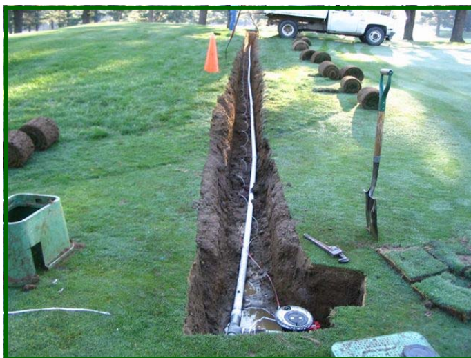
Steve and members of the superintendent's staff install a new sprinkler head between the cross bunker and the third green (above and below)
