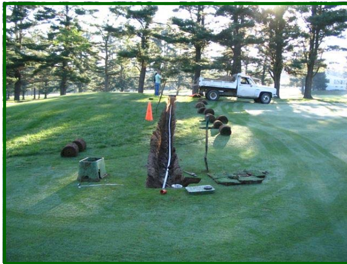
Steve and members of the superintendent's staff install a new sprinkler head between the cross bunker and the third green (above and below)
